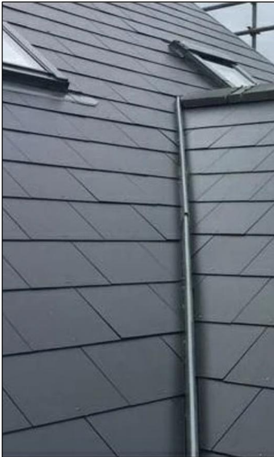
Roof Tiles Cembit Jutland Fibre Cement Slate Graphite 600x300mm
